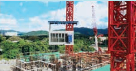
Stage 4 On-site installation of MiC modules and jointings
